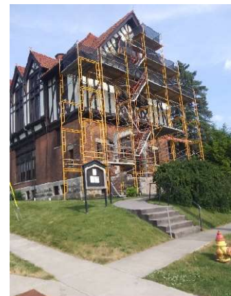
Scaffolding in place 6/15/23
