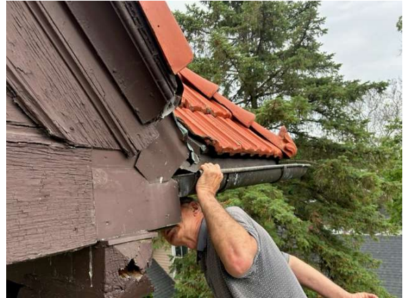
South Side looking at roof edge and fascia construction – 6/15/23
