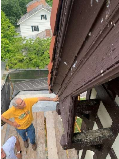
North Side looking down along existing roof edge and fascia construction – 6/20/23
