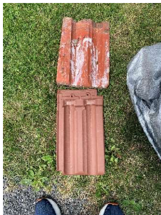
Existing tile from peak upper and new tile lower – 6/20/23
