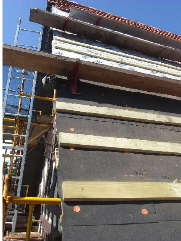
SOUTH FACE DETAIL SHOWING NEW PURLINS AND NEW MOISTURE BARRIER
