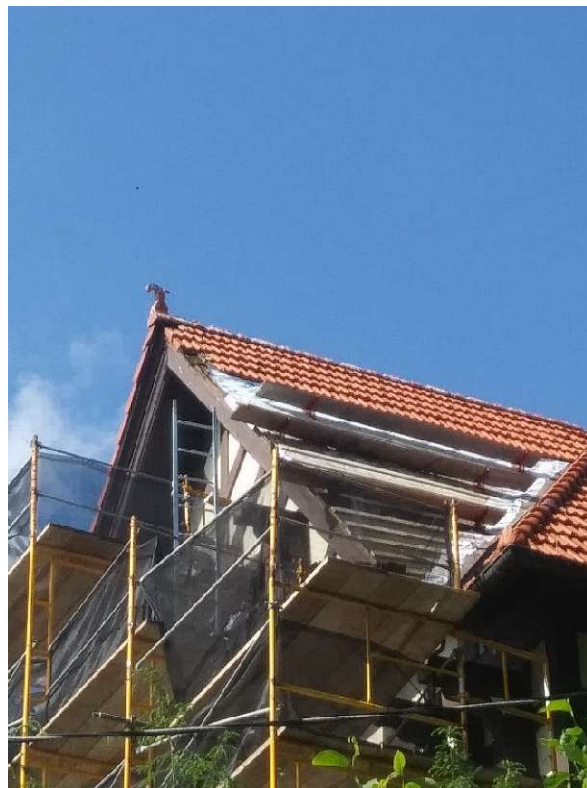
SOUTH FACE PROGRESS – BLUE SKY TOO
