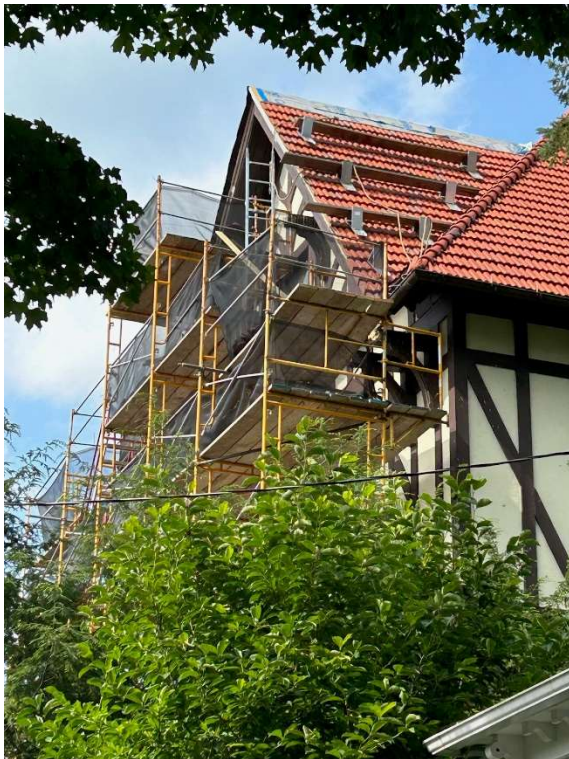
SOUTH FACE LOOKING UP RAKE
