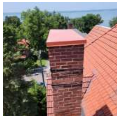
Chimney after – looking west
