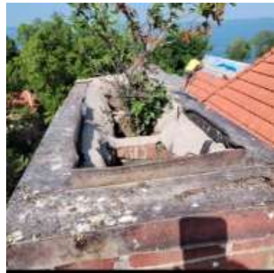
Chimney before – looking west
